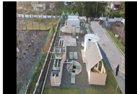
1 MLD CSTP at Padanappalam, Kannur
