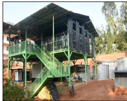
1 MLD STP at Kozhikode medical College
