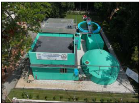
360 KLD STP at General Hospital, Thrissur
